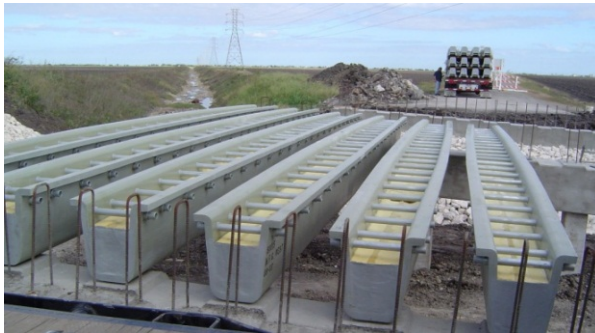
Fig. 16. Hybrid FRP/Reinforced Concrete Bridge Girders Evaluated with Acoustic Emission (after Ramirez et al., 2009)
