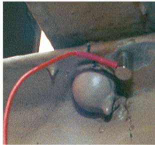
Fig. 2. AE Sensor on Brooklyn Bridge Floor Beam
