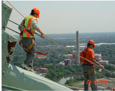
Fig. 6. Installing Sensors for Long Term Monitoring of a Suspension Bridge Cable
